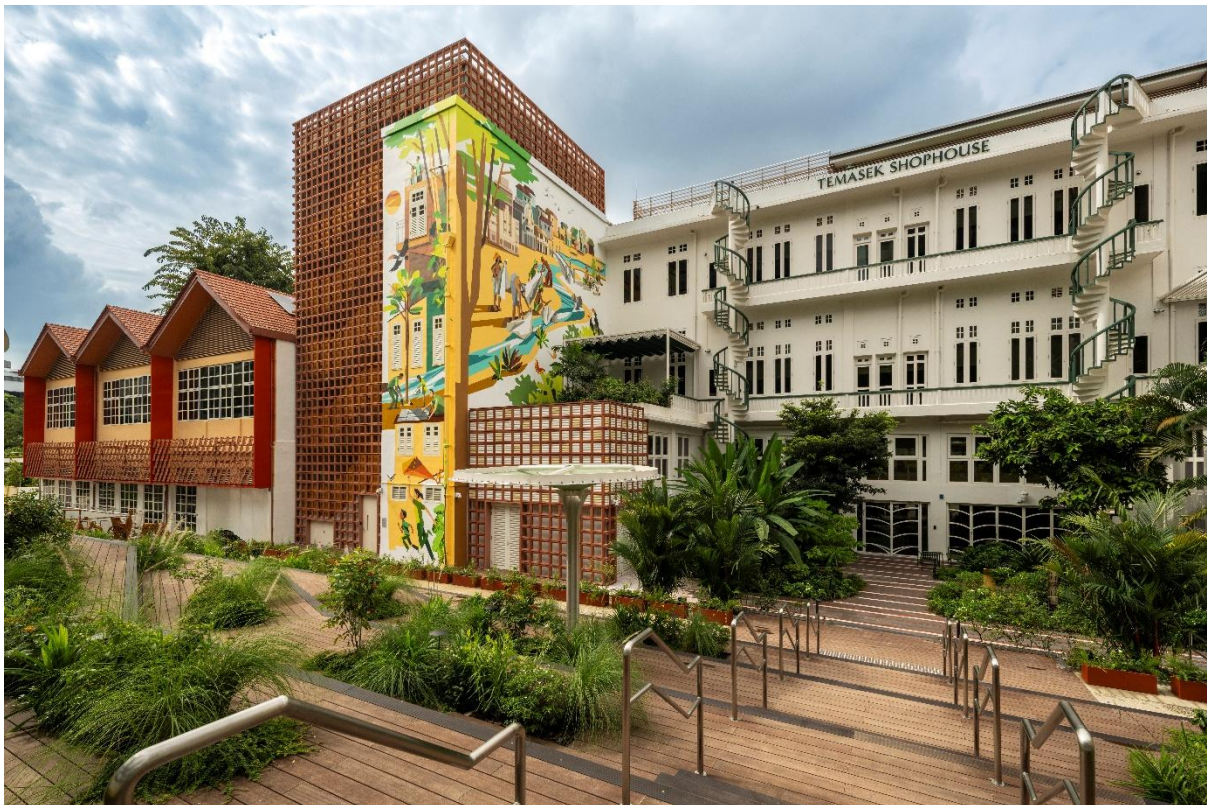
View of the Outdoor Community Space at Temasek Shophouse. Image © Darren Soh
